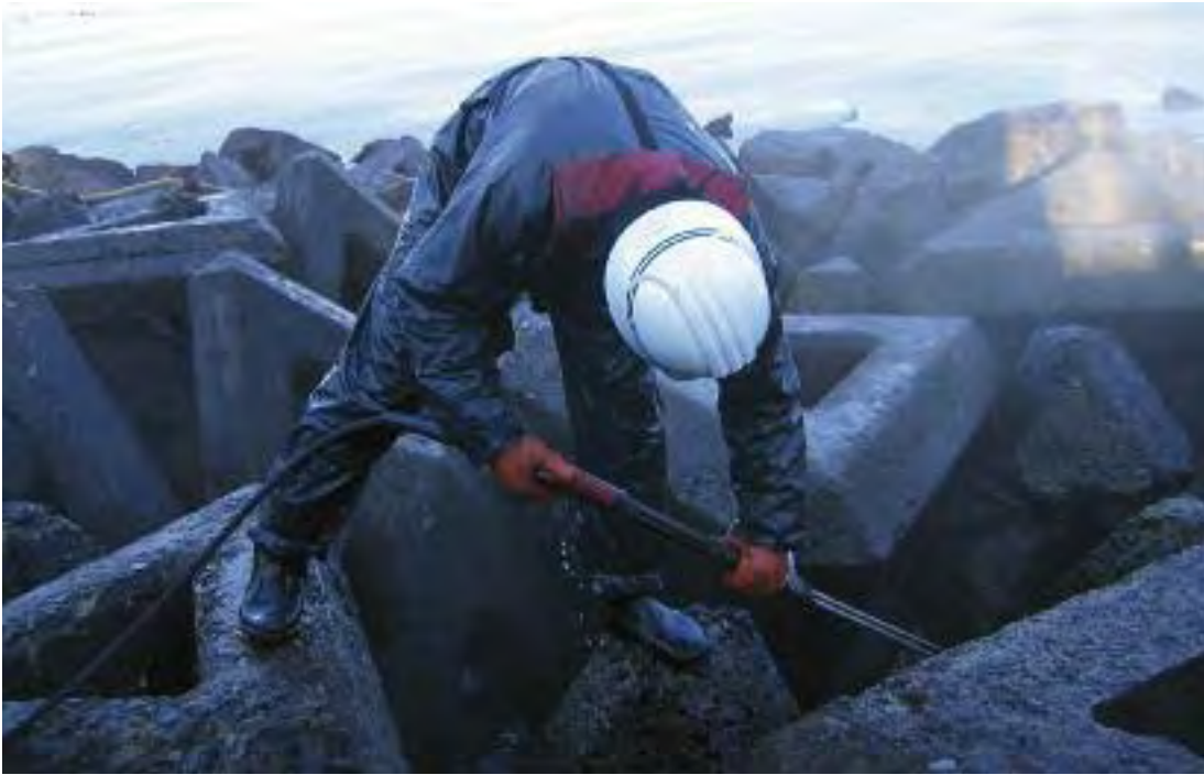
Shosei Maru: Boat pier being cleaned using a high pressure gun spraying hot water and chemical solvent
