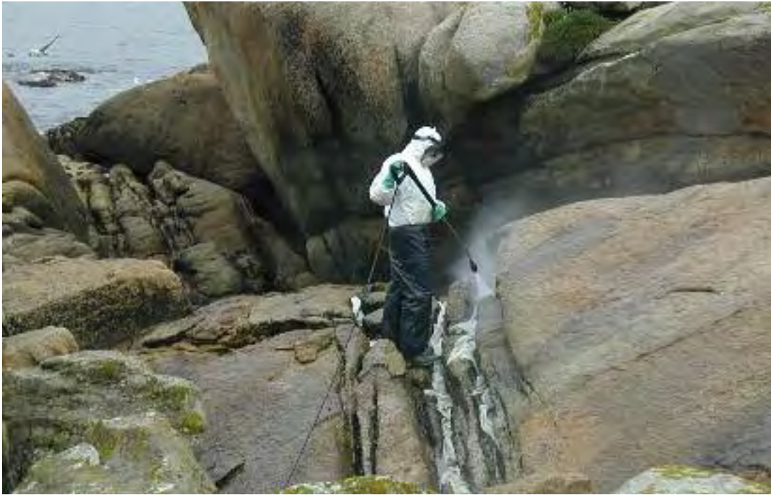
Prestige: Rocky shorelines were cleaned using high pressure washing
