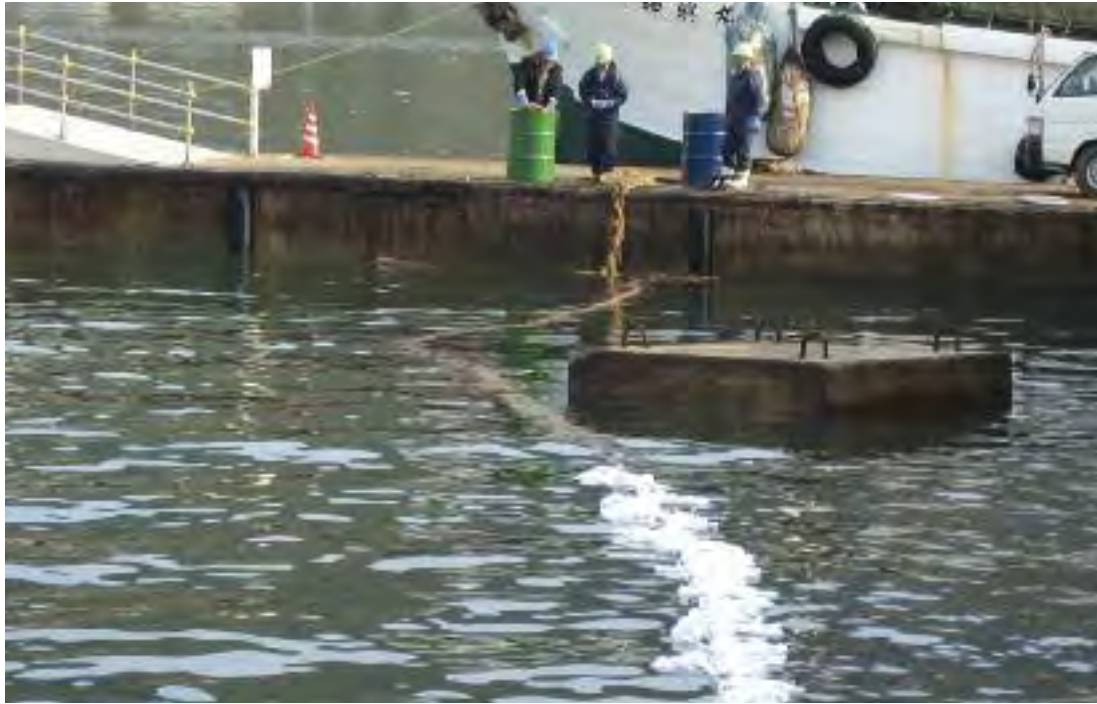
Shosei Maru: Deployment of sorbent boom
